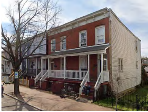
332/334 S Laurel St - Semibasement + Porch
