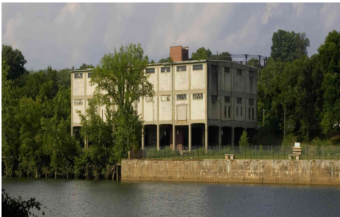
Intermediate Terminal Wharf adjacent to Warehouse #3
