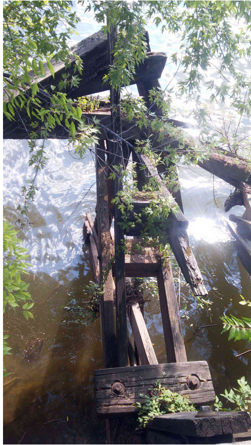
Wooden pylons extant on Intermediate Terminal Wharf structure.
