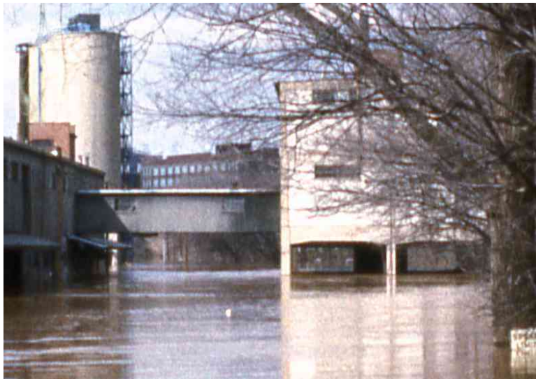
The innovative construction of the Terminal Warehouse #3 (right) on concrete reinforce piers provided protection from floods. (Source: VCU Archives 1979)
