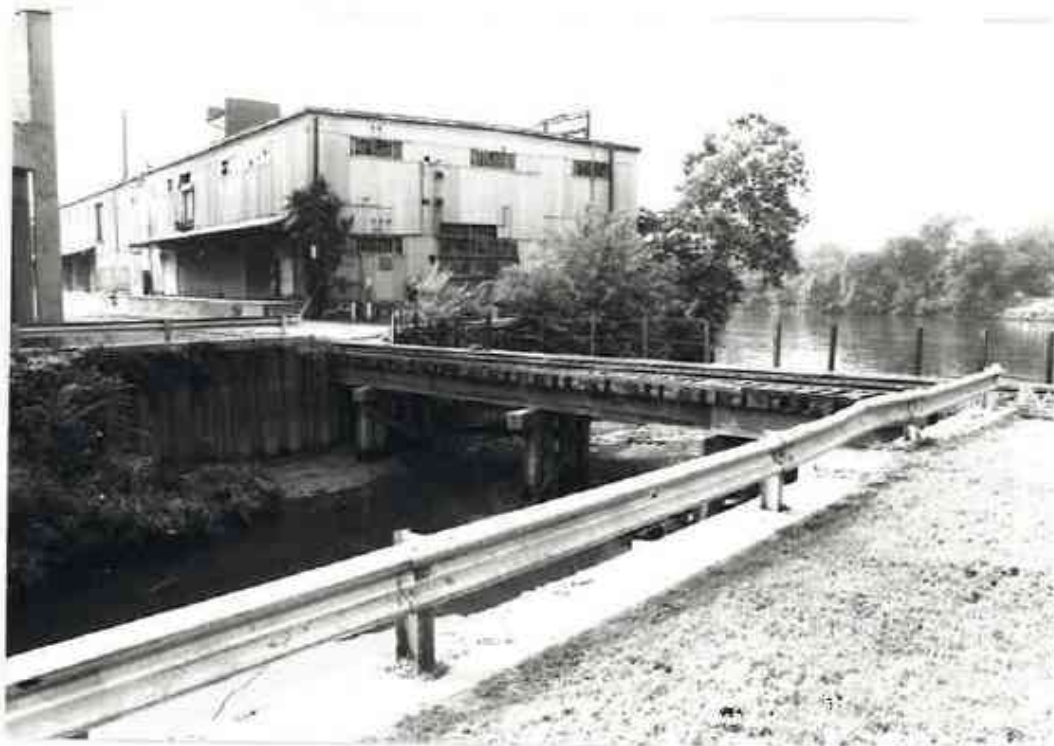
1938 Water Street Bridge over Gillies Creek adjacent to the Terminal (determined to be potentially eligible for the NRHP) and 1930s (?) former railroad bridge now converted to bicycle path. (Source: VDHR)
