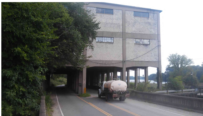
The Terminal's construction of piers resulted in a striking, iconic building, known as the “tunnel” building. This significant design feature will become more important as global warming results in more urban flooding.
