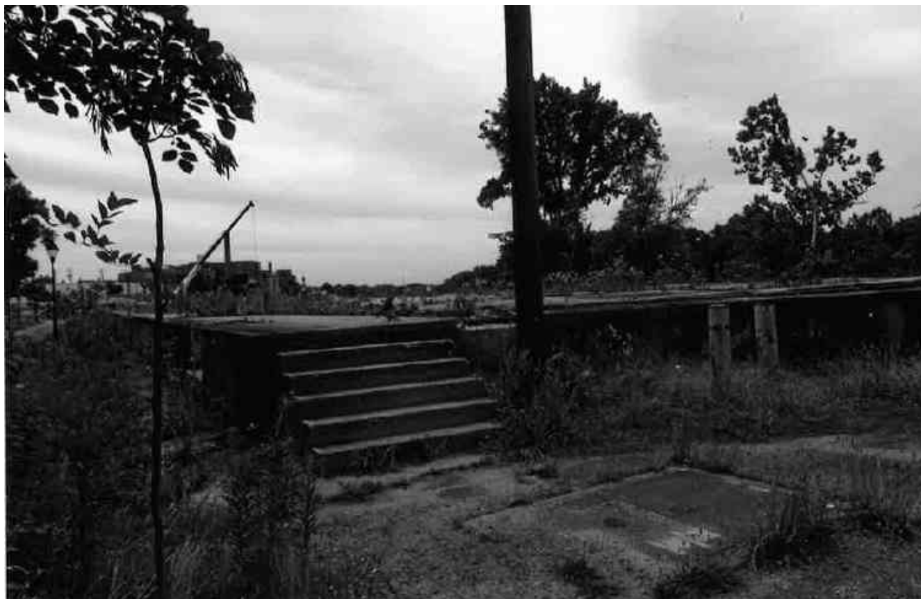
Concrete foundation pad for Warehouse No. 1 and 2, in 2016 VDHR photo. The recent removal of the foundation pads without the required Section 106 review constitutes anticipatory demolition and should be of grave concern to the Advisory Council for Historic Preservation. (Source: VDHR file #127-6975)
